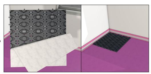
Place the second Profix® Panel with the arrow heads facing to the left and engage them into the gates along the right hand edge of the first panel. Peel off the backing sheet on the second panel to expose the adhesive and stick it down.
